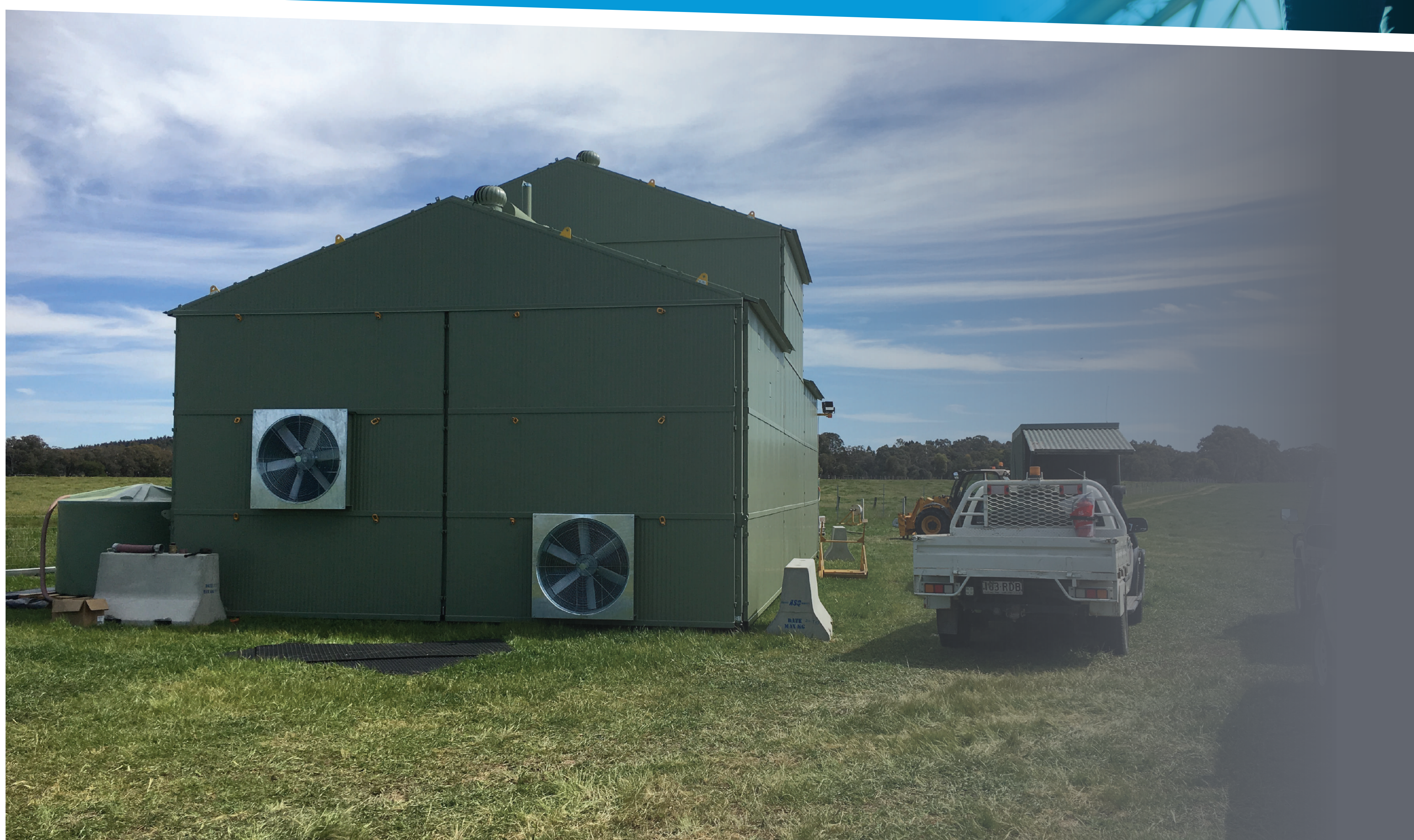
Left: Drill rig enclosed in acoustic shed.
