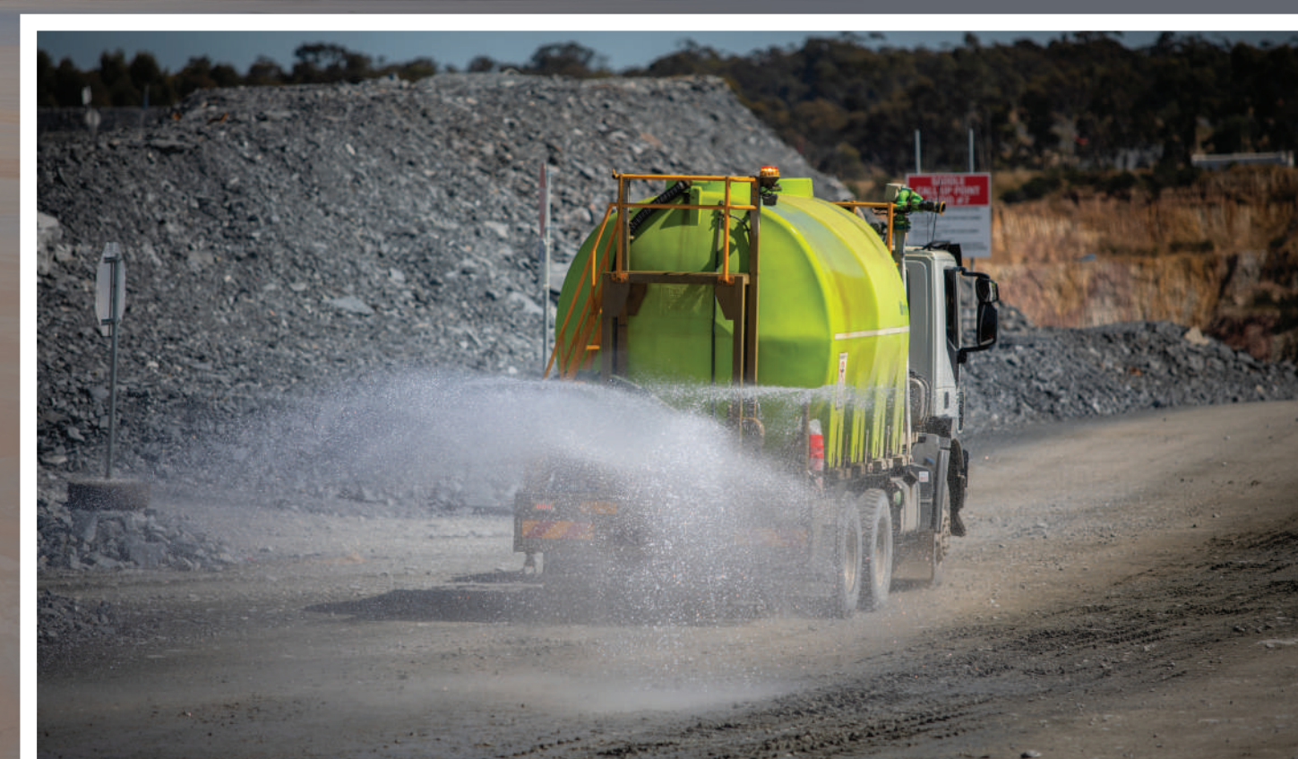
Applying water to reduce dust on unsealed roads
